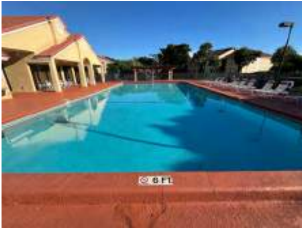
The swimming pool and spa located at the clubhouse were recently repaired/refinished. Pool refinishing is normally needed about every ten years. Although we allow for this work to occur on that schedule, the decision to whitecoat should be evaluated annually and conducted when necessary. Sundeck coating at pool deck was also replaced.
