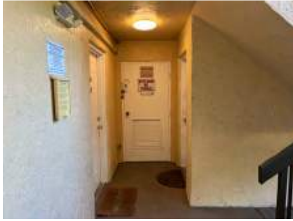
...as is replacement of common utility room doors.
