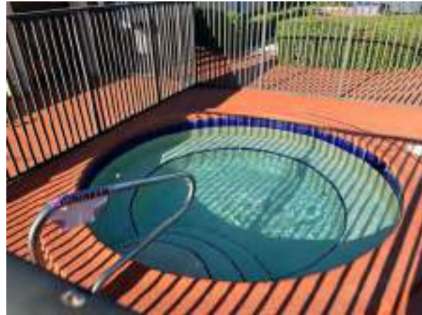
The swimming pool and spa located at the clubhouse were recently repaired/refinished. Pool refinishing is normally needed about every ten years. Although we allow for this work to occur on that schedule, the decision to whitecoat should be evaluated annually and conducted when necessary. Sundeck coating at pool deck was also replaced.
