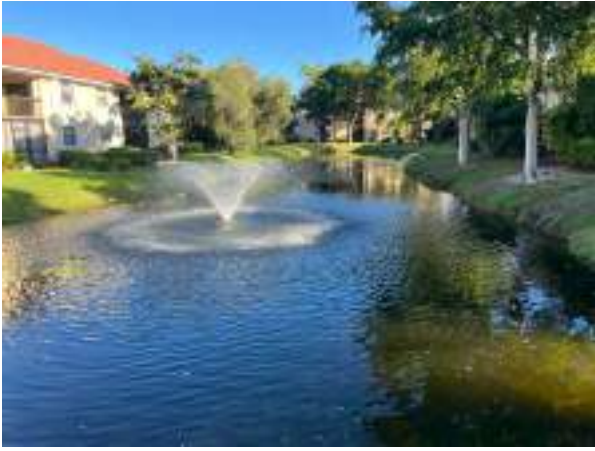
Fountains and power units need replacing when they fail.
