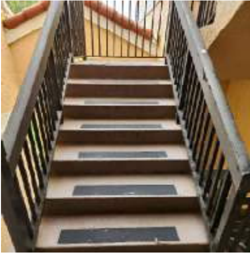
Railings (Good condition)
