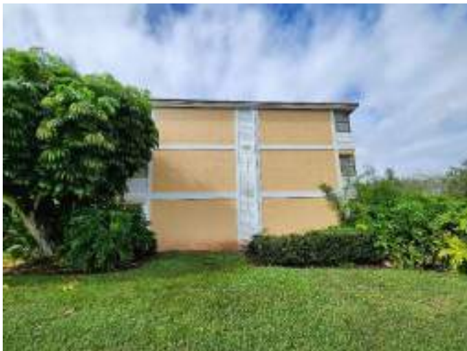
Side of building (North elevation)
