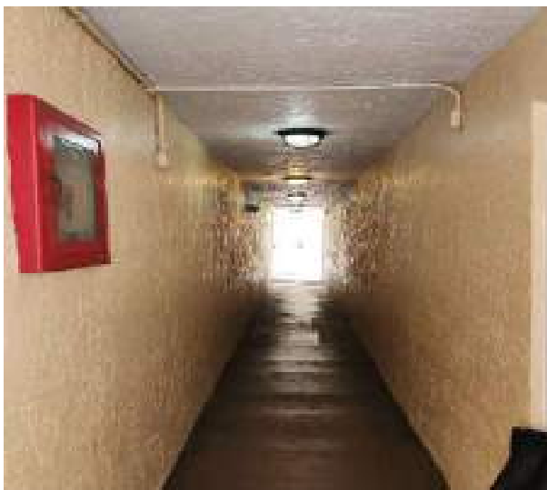
Building egress illumination
