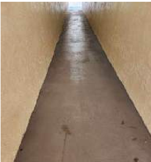
Corridors (Good condition)
