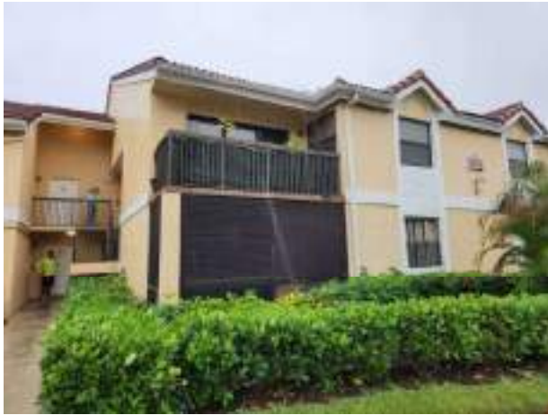
Front of Building (West Elevation)
