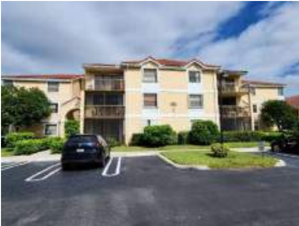
Front of Building (South Elevation)
