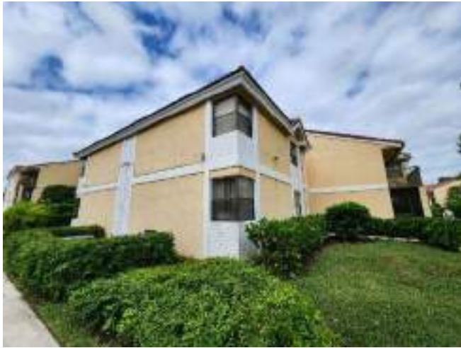
Side building (South elevation)
