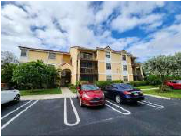
Front of Building (West Elevation)
