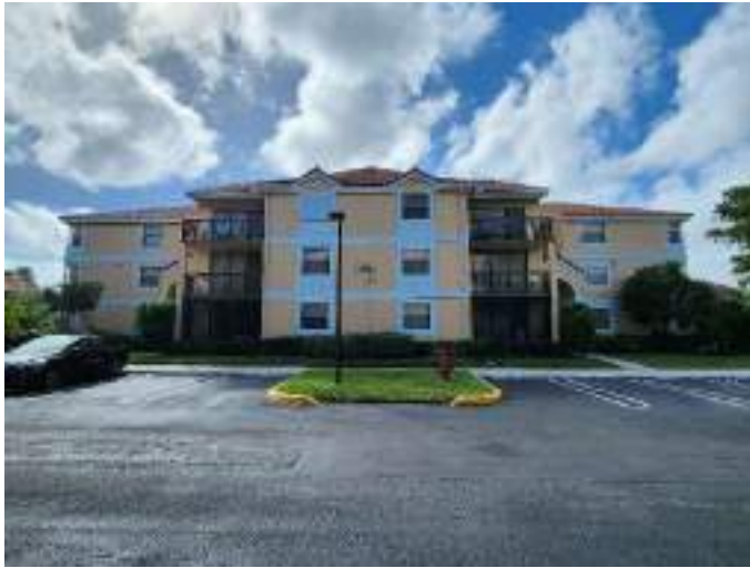
Front of Building (East Elevation)
