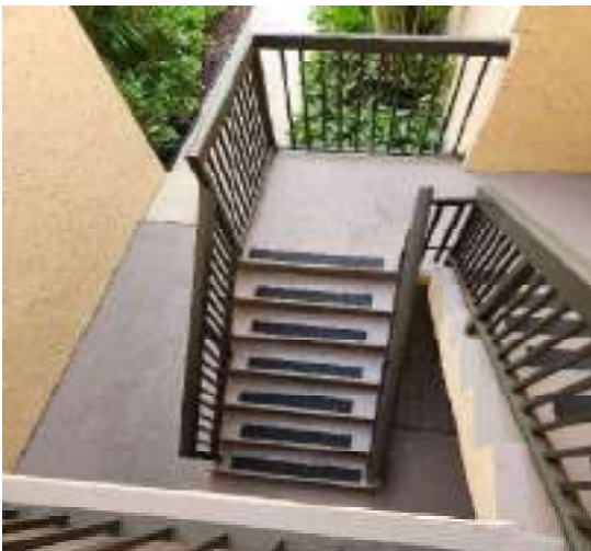
Stairs and railings (Fair condition)
