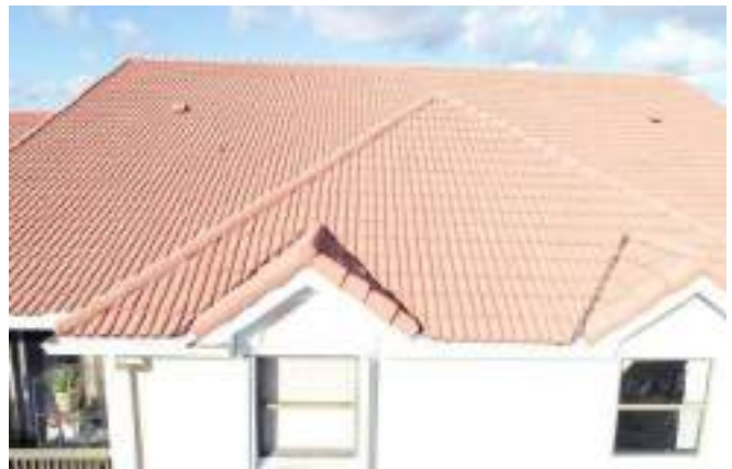
General Roof Pictures
