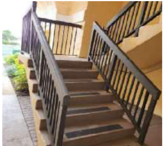
Railings (Good condition)
