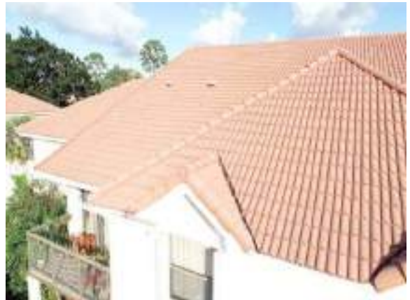
General Roof Pictures
