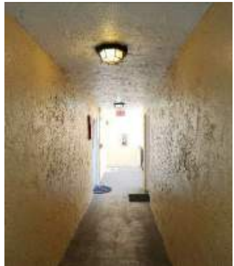
Building egress illumination
