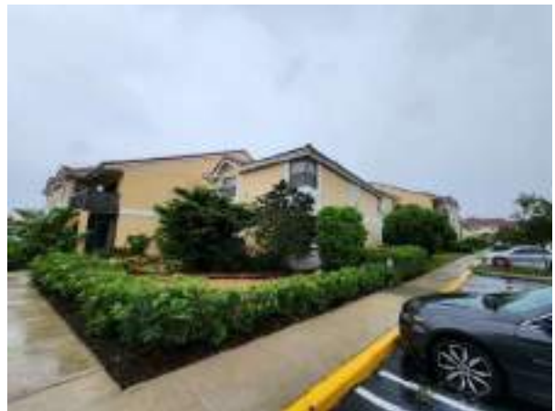
Side of Building (East Elevation)
