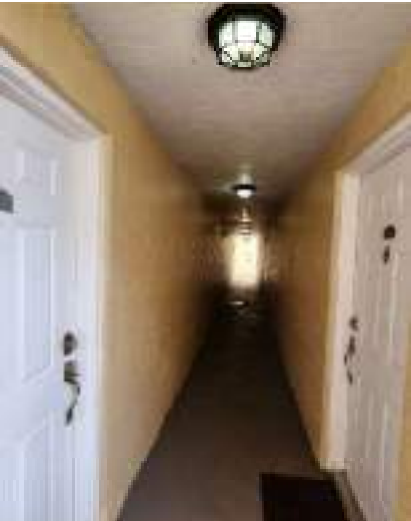
Building egress illumination
