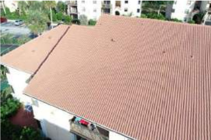
General Roof Pictures
