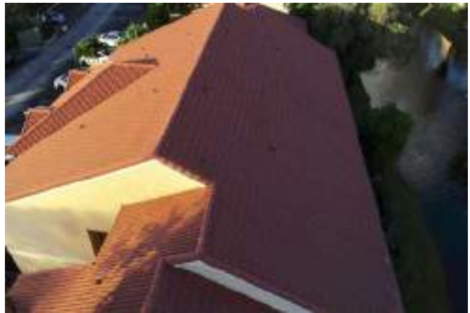
General Roof Pictures
