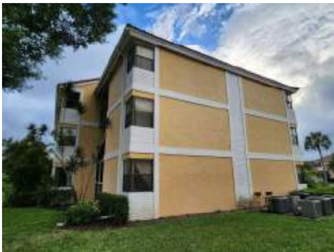
Side Building (North Elevation)
