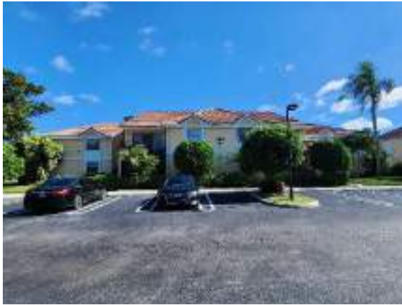
Front of Building (West Elevation)
