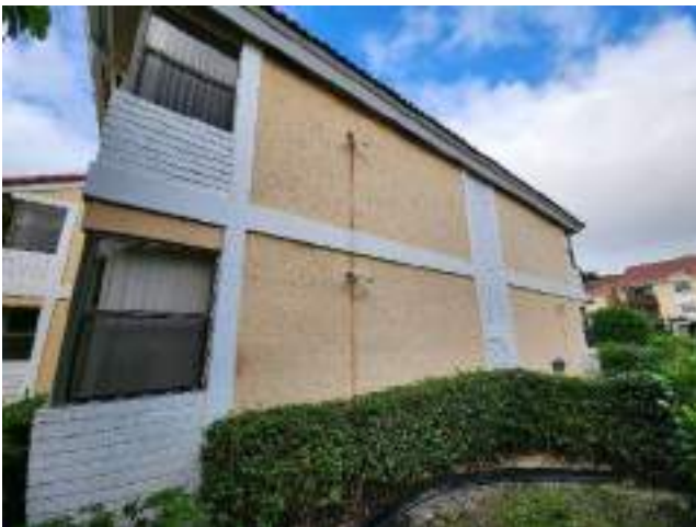
Side Building (North Elevation)
