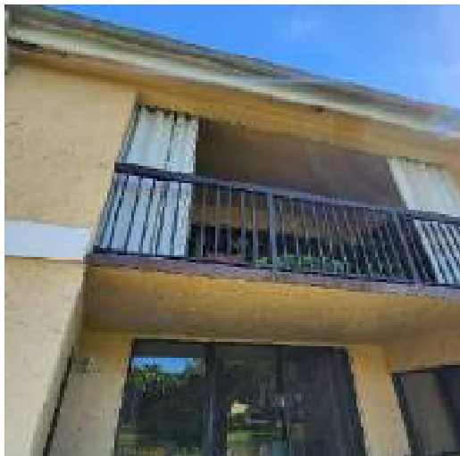
Balconies (Fair condition)
