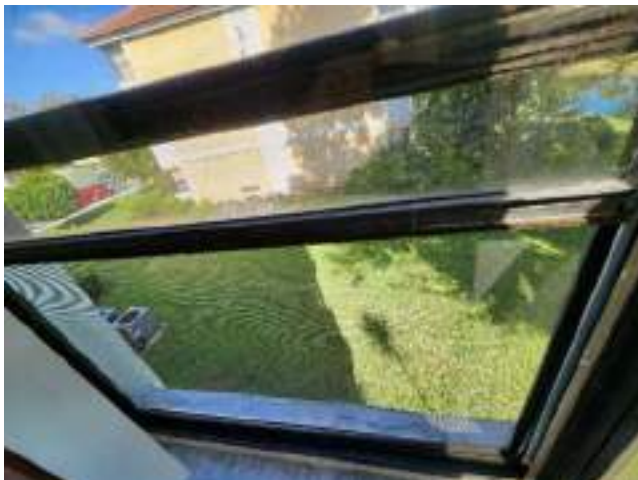
Exterior Windows (Good condition)
