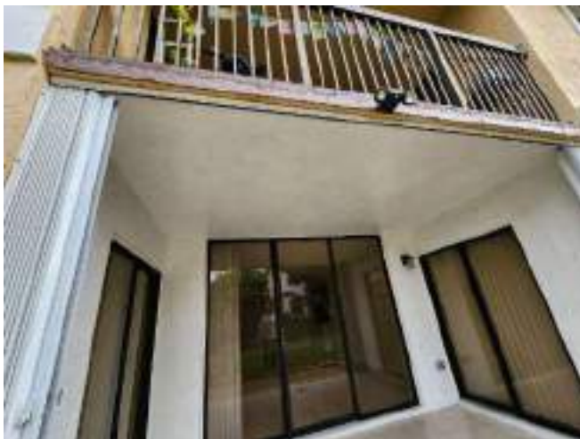
Railings and balconies (Good condition)
