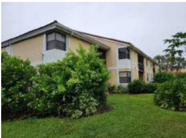
Rear of Building (North Elevation)
