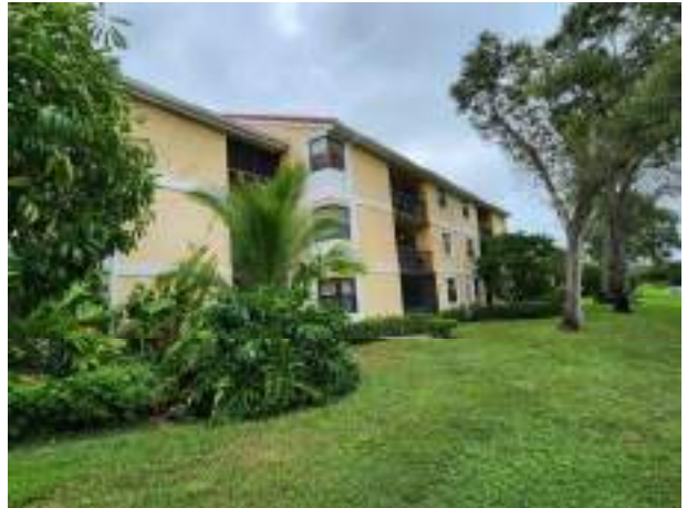
Rear of building (West elevation)
