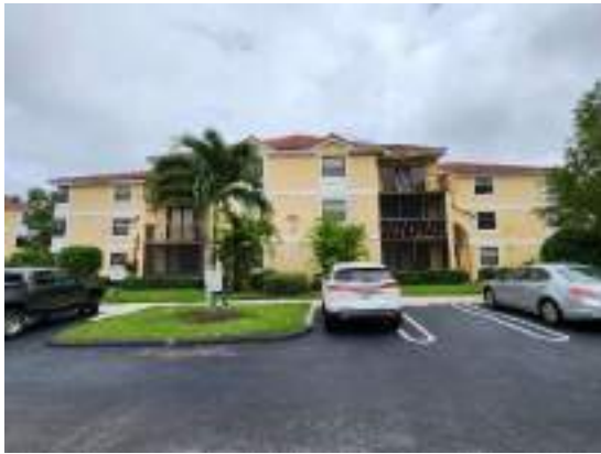
Front of Building (West Elevation)
