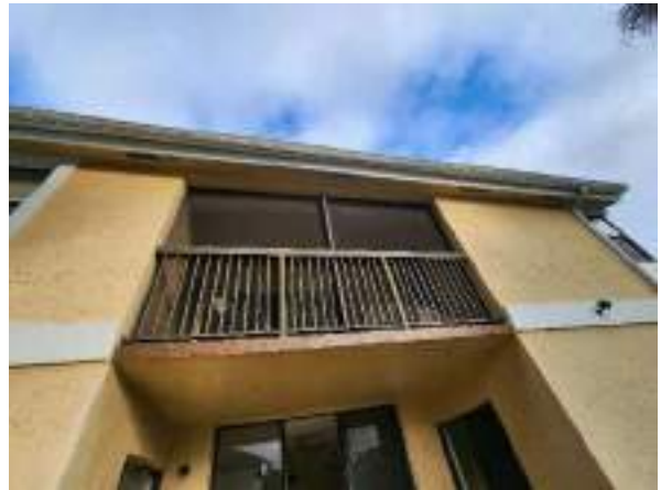
Railings and balconies (Fair condition)
