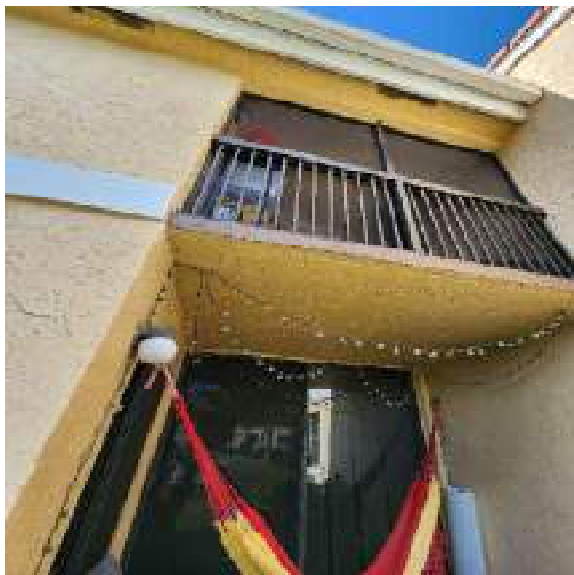
Balconies (Fair condition)
