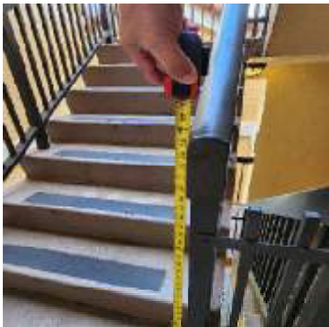
Stairs and railings (Fair condition)
