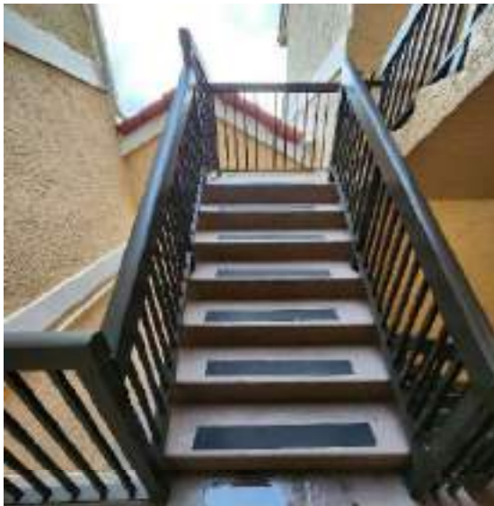
Stairs and railings (Fair condition)
