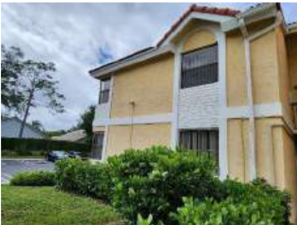
Side Building (North Elevation)
