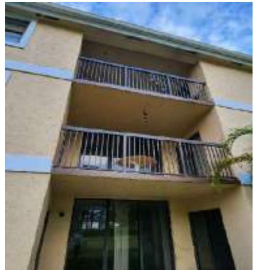
Railings and balconies (Good condition)
