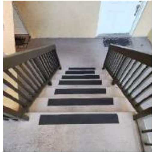
Stairs and railings (Fair condition)
