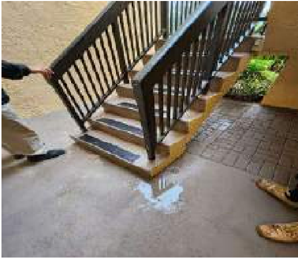
Railings (Good condition)
