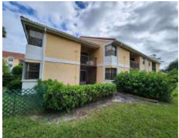
Rear of building (West elevation)
