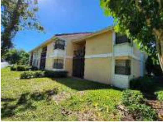
Rear of building (North elvation)
