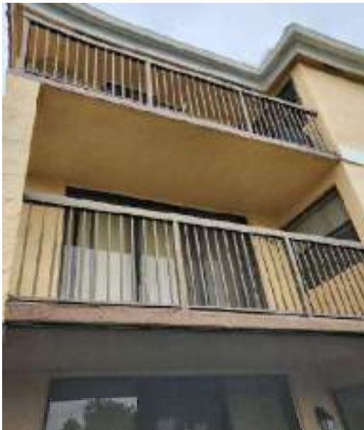
Railings and balconies (Good condition)
