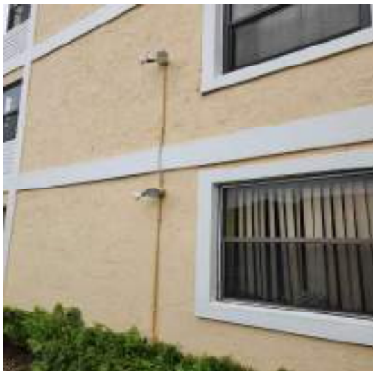
Rear of Building (North Elevation)
