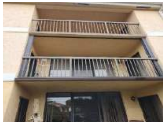
Balconies (Good condition)
