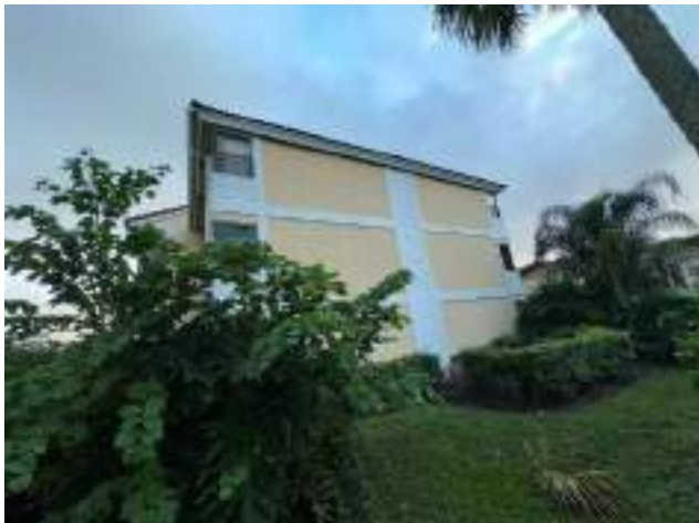
Side of building (South elevation)
