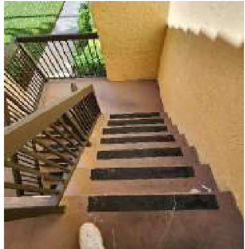
Stairs and railings (Fair condition)
