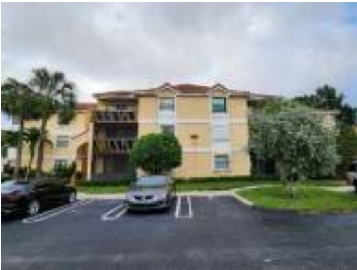
Front of Building (East Elevation)
