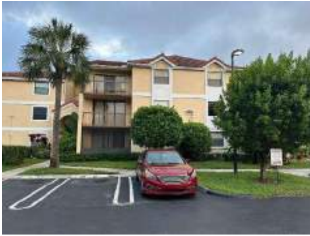
Front of Building (West Elevation)
