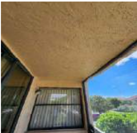
Balconies (Fair condition)
