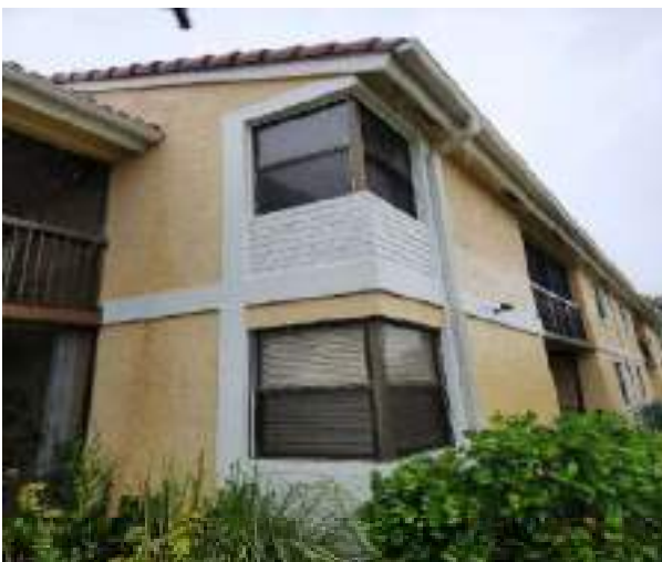
Exterior Windows (Good condition)
