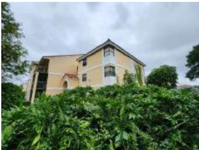
Side Building (North Elevation)
