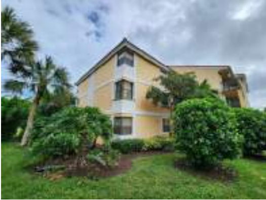
Side building (South elevation)
