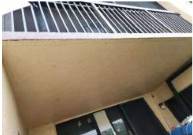
Balconies (Good condition)
