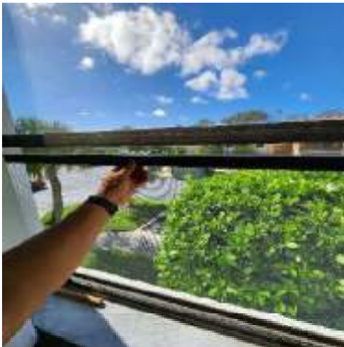
Exterior windows (Fair condition)
