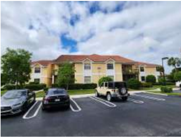
Front of Building (East Elevation)
