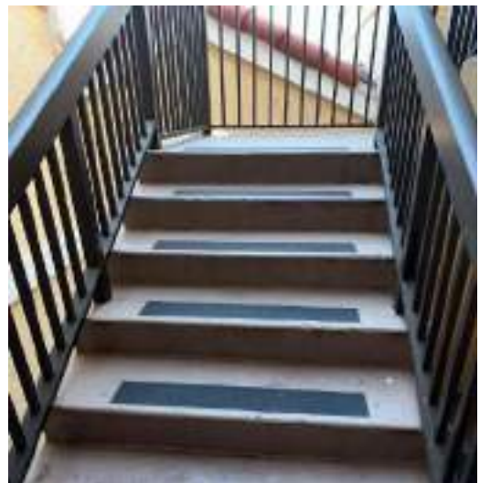
Stairs and railings (Fair condition)
