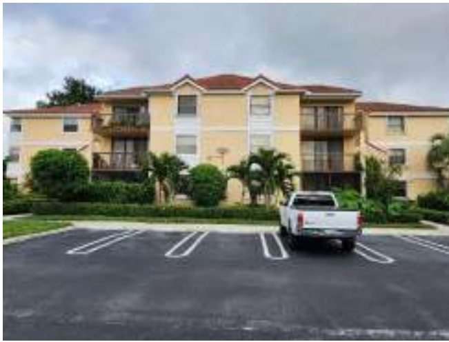
Front of Building (West Elevation)
