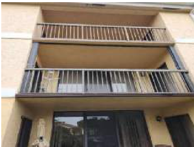
Balconies (Good condition)
