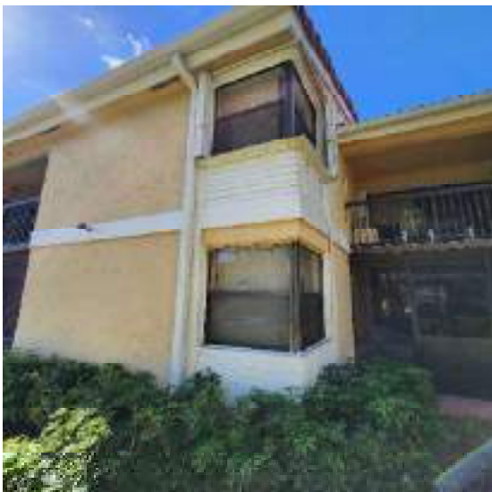
Side of building (South elevation)
