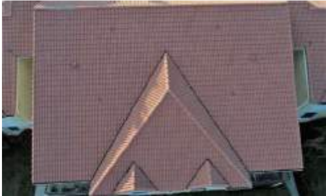
General Roof Pictures
