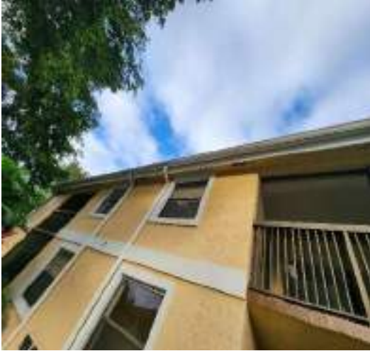
Rear of building (West elevation)
