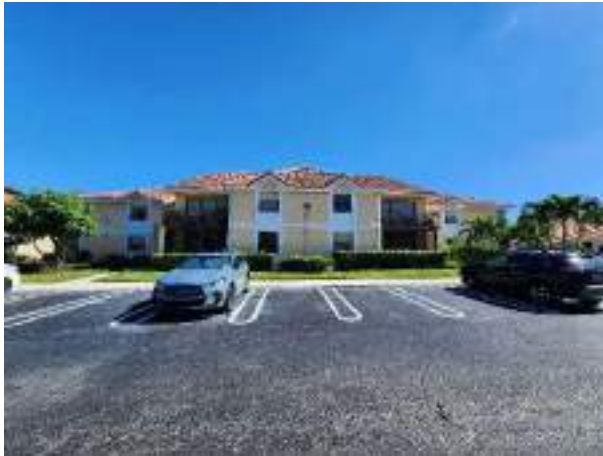
Front of Building (West Elevation)
