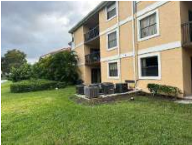
Rear of building (West elevation)
