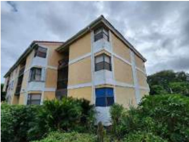
Rear of Building (North west Elevation)
