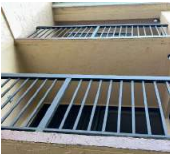
Balconies (Fair condition)
