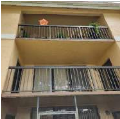
Balconies (Fair condition)
