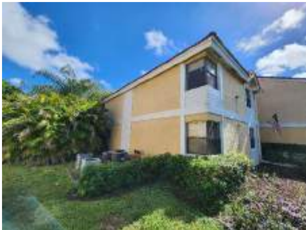
Side of building (South elevation)
